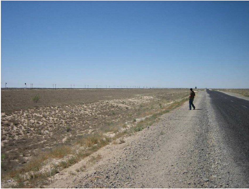
Figure 11: Over long distances M32 as well as the railway, power lines and pipelines run parallel to each other, thus forming a wider “infrastructure corridor”.
