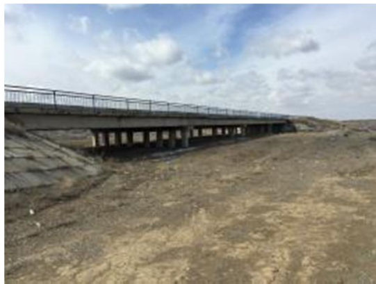
Photo 12: Bridge on Road
