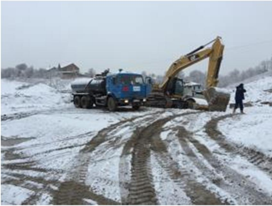
Photo 1: Almaty /Kapshagay Road Works
