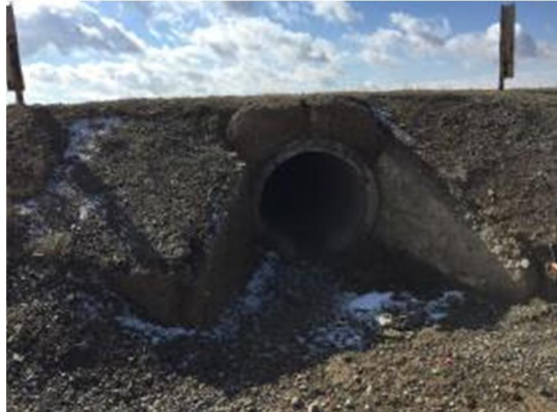
Photo 8: Culvert under Road
